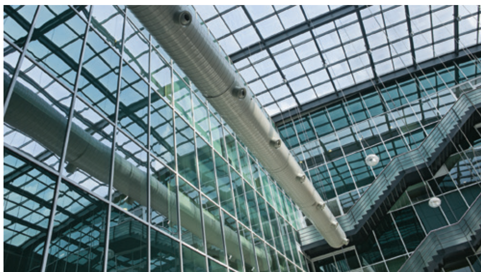
Figure 1: The curtain walls and ventilation ducting shown in this image take advantage of aluminum's inherent properties: lightweight, strong, flexible, and long-lasting.
