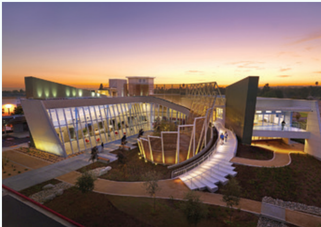
Figure 4: Frontier Project, Rancho Cucamonga, California. Energy efficiency and thermal performance were key considerations in the design of this LEED® Platinum certified building. A north-facing glass wall provides daylight while the double-paned glass with a low-E coating, supported by high-strength, low-weight aluminum frames, reduces radiant heat transfer.
