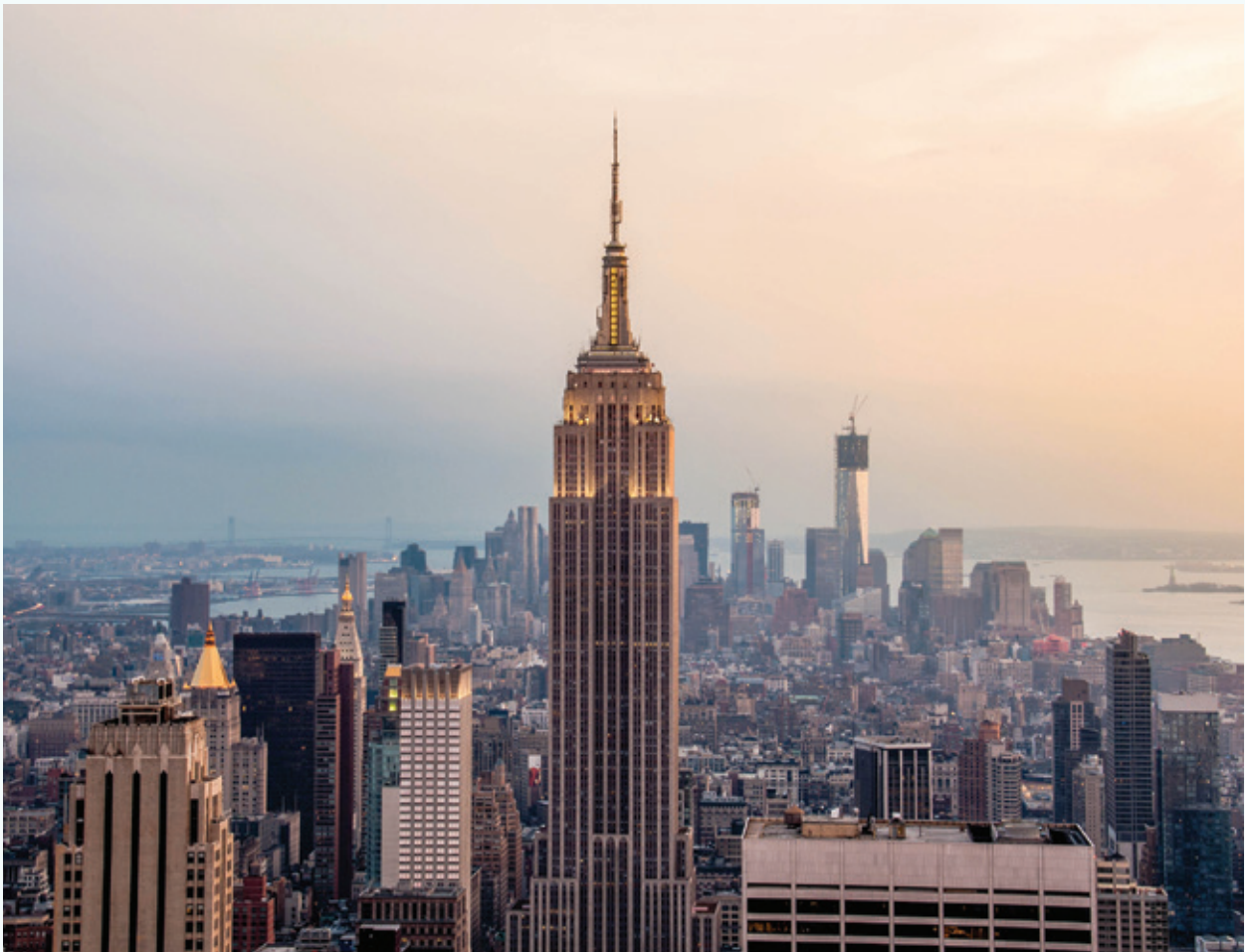
Figure 7: An American cultural icon, the Empire State Building, constructed in 1930-1932, was the first building to make major use of aluminum components and fabricated structures.
