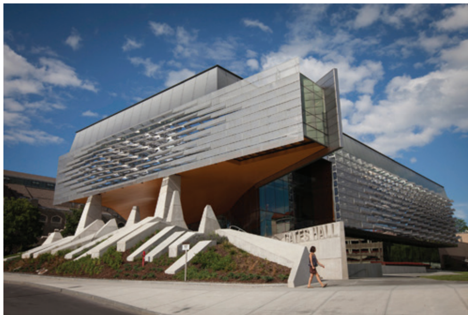
Figure 5: Gates Hall, Cornell University, Ithaca, New York. To meet the needs of the students and faculty, it was vital for the building to feature copious amounts of natural light and open spaces. The building was designed to incorporate a 35,000 square foot aluminum curtain wall, offering sprawling views of the picturesque campus.
